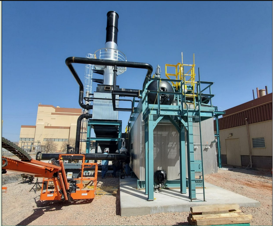
A $5 million LEDA Grant from NMEDD allowed McKinley Paper to add a new boiler and associated equipment to generate the steam it needs to produce cardboard.
